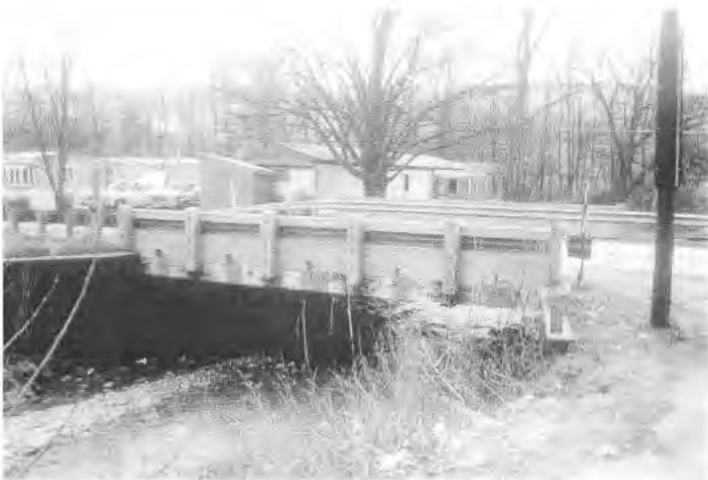
(a) End view of the Angelica Bridge showing the railing unit.
