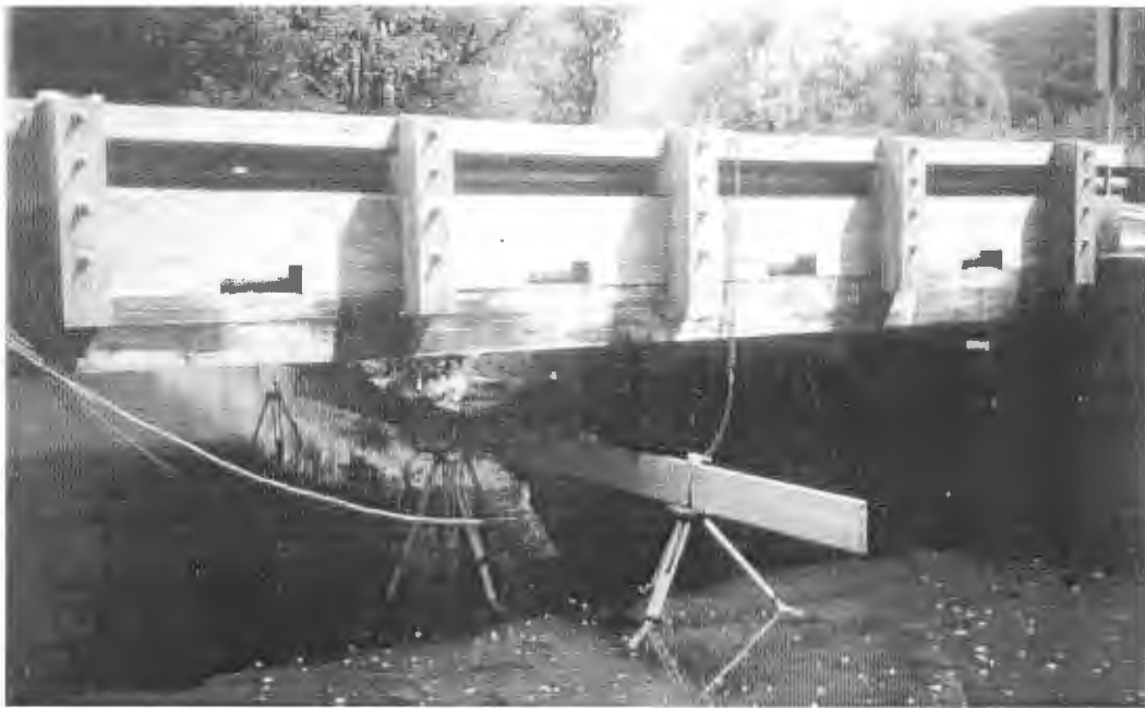
(b) End view of the Bolivar Bridge.
