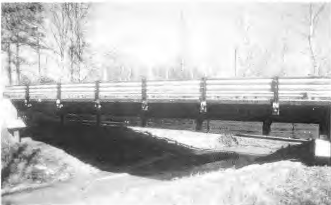
(b) End view of the Chambers County Bridge showing the girders.
