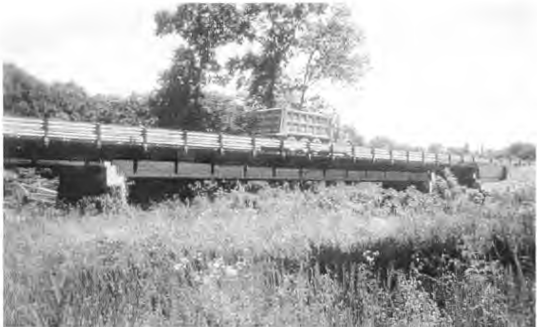
(b) End view of the Wittson Bridge showing the girders.
