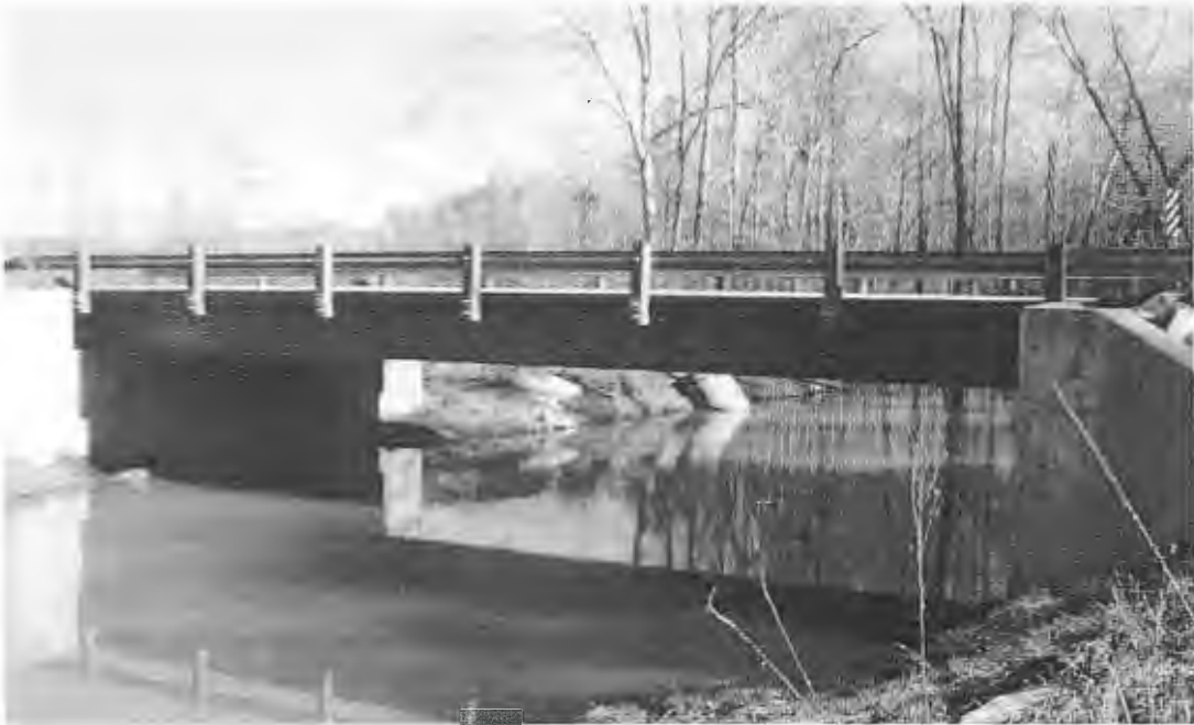
(a) Single span glulam girder bridge.
