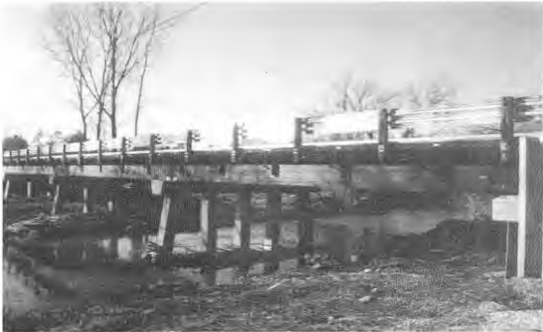
(b) Multi-span glulam girder bridge.
